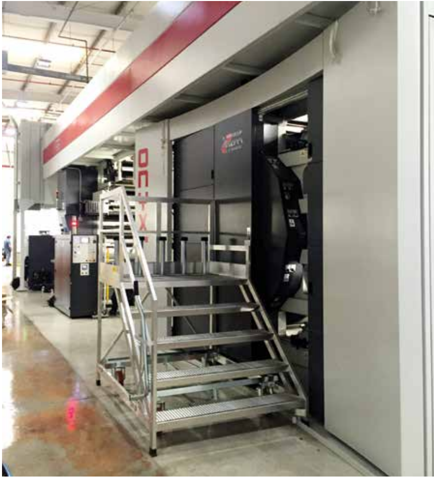
Poly Print installed a new 10-color flexo press in May 2016, bringing its number of wide web flexo presses to three.
